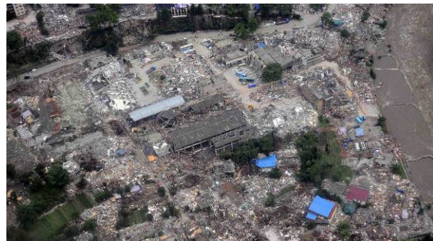
Fig 2. A school in Wenchuan after earthquake (www.news.sohu.com)
